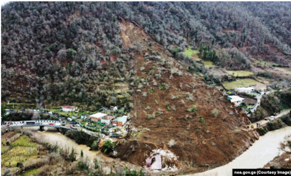
Fig. 2. Landslide in Nergeeti [https://www.radiotavisupleba.ge/a/32895673.html].
