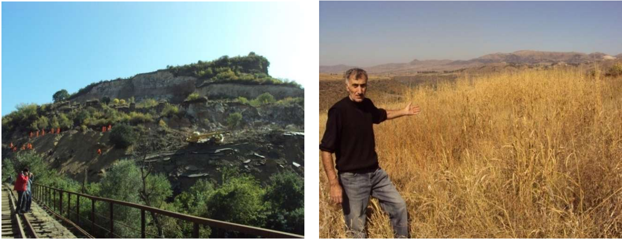
Fig. 1. Overview of Ayrum landslide-collapse area (the basalt cover is destroyed). On the site, above the collapse, the ground is water-saturated, wetlands.
